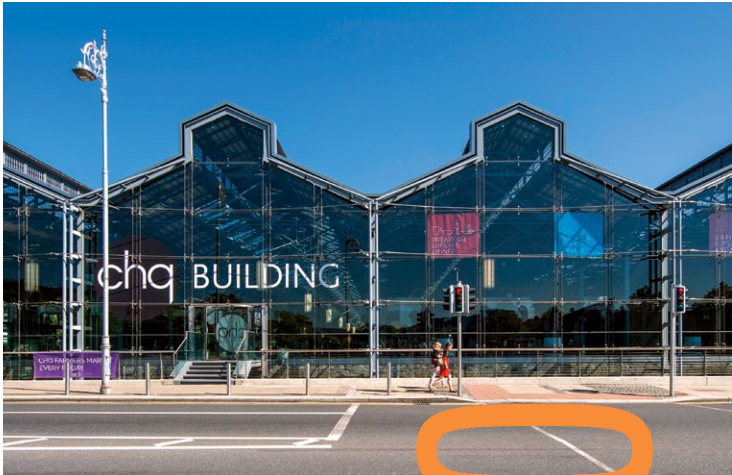
CHQ Dublin, 1 Custom House Quay
